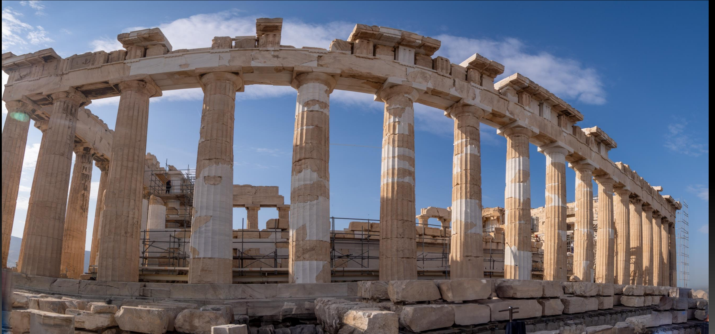
Still Under Construction Submitted by Walt Lyons
