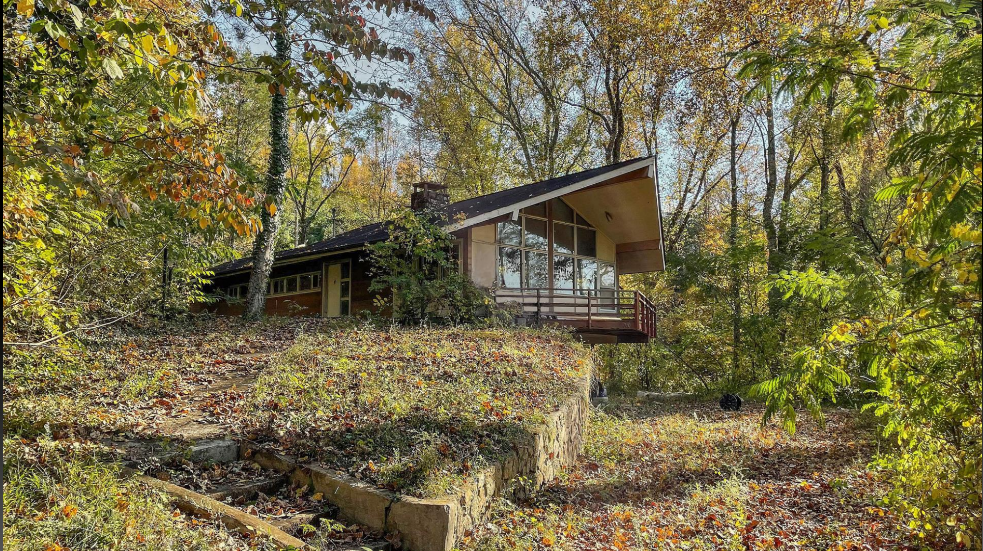
Abandon House by Ed Ogle
